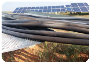
Improper Cable Routing
