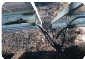
MC4 Connectors / Y junctions ... poor crimping ?
