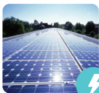
Solar Photovoltaic (PV)
