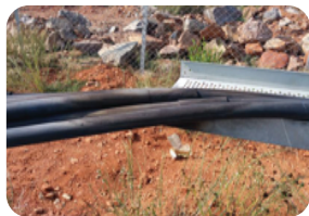
Cable Heating up
