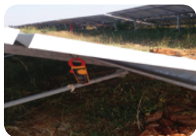
Ground clearance issues
