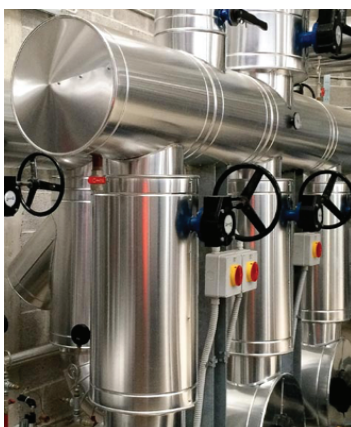
Proper Insulation at Steam Distribution
