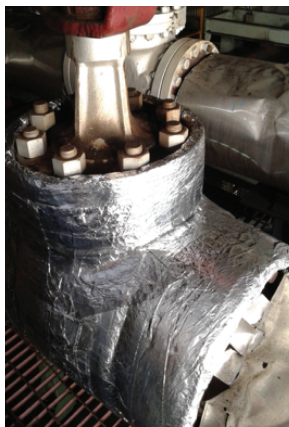
Proper Insulation at Valves
