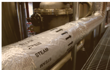
Proper Insulation at Steam Lines
