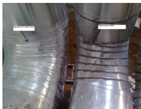
Proper Insulation at Bends
