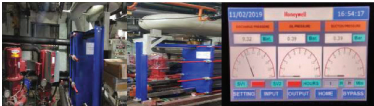
Figure 27: Post Implementation – Direct Cooling Method
