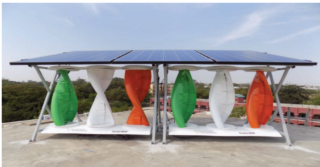
Figure 52: Solar wind hybrid system
