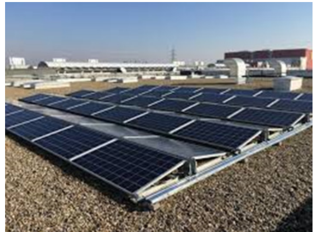
Figure 21 : Solar PV installation
