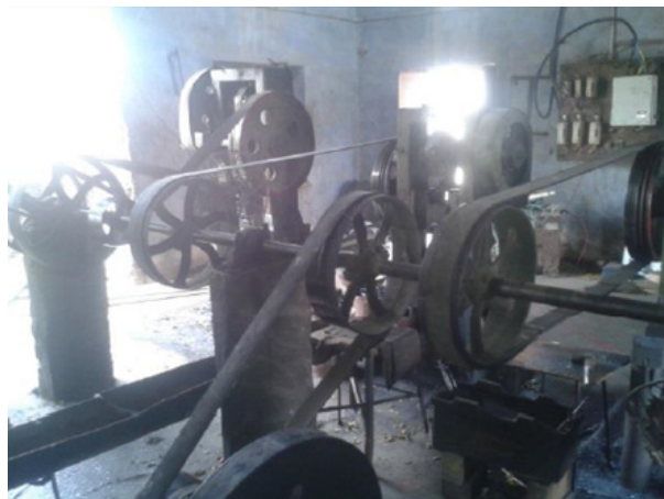
Figure 24: Inefficient belt and pulley drives
