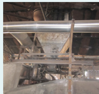
Modified pulverized coal feeding system at TK Steel
