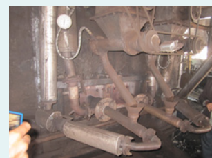
Pulverized coal swirl burner
