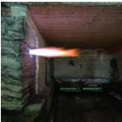
Figure 42: High Velocity Burner with Flame
