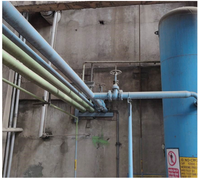
Figure 29: Existing compressed air piping
