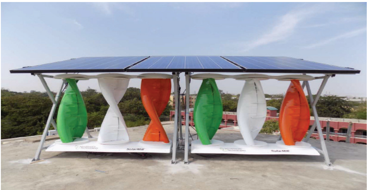
Figure 38: Solar-wind hybrid system
