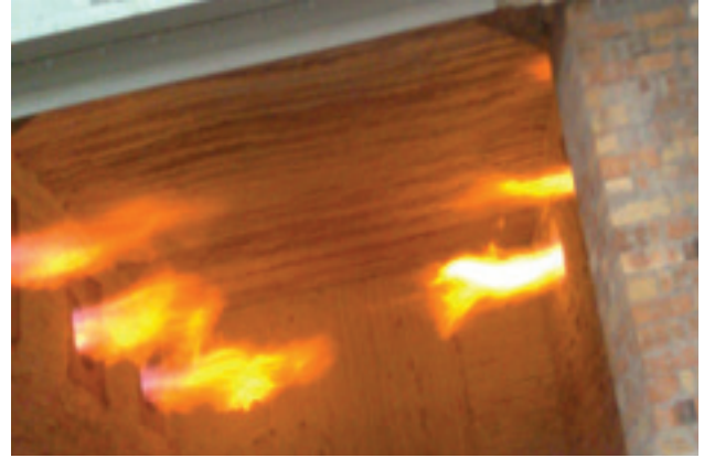
Figure 44: Improper air to fuel ratio
