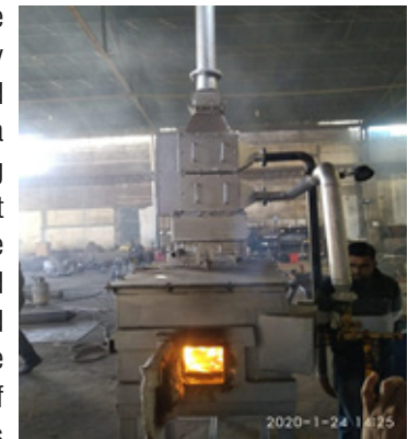
Figure 5: Energy efficient FO fired forging furnace
