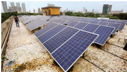
Figure 15: Roof Top Solar PV Installation
