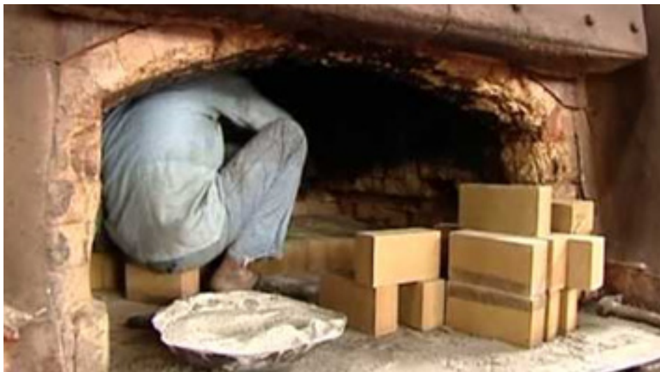
Figure 21: Heat treatment furnace veneering process
