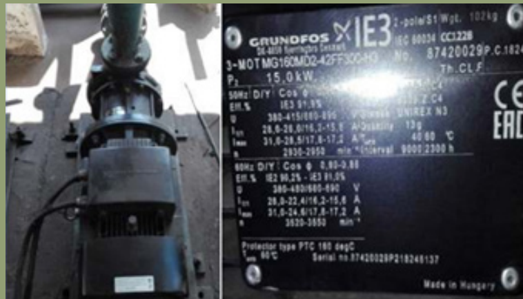
New EE Pump at Integra Automation
