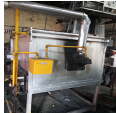
Figure 6: LPG fired forging furnace
