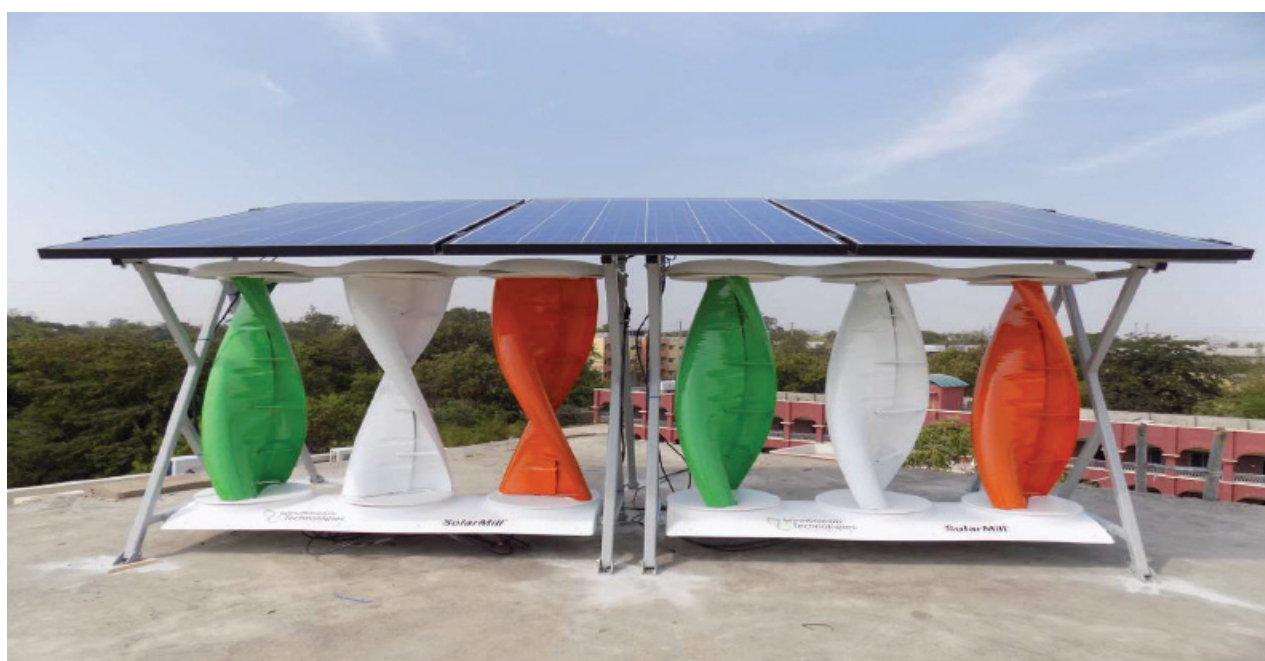
Figure 43: Solar wind hybrid system
