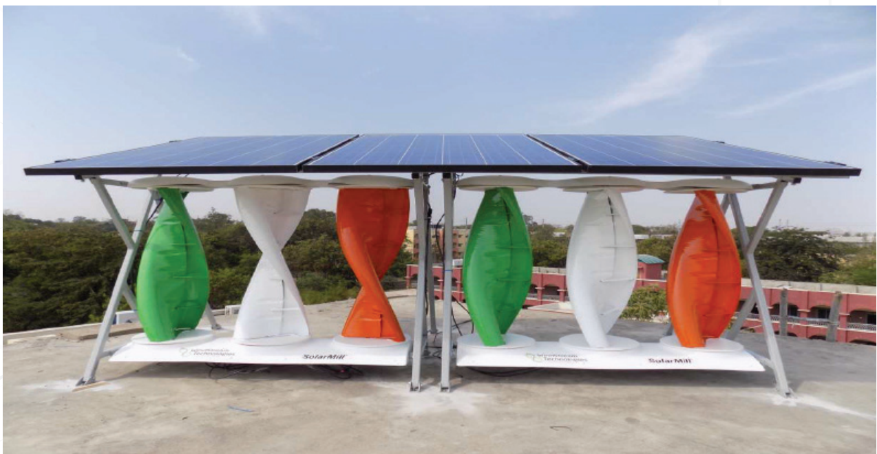
Figure 32: Solar wind hybrid system
