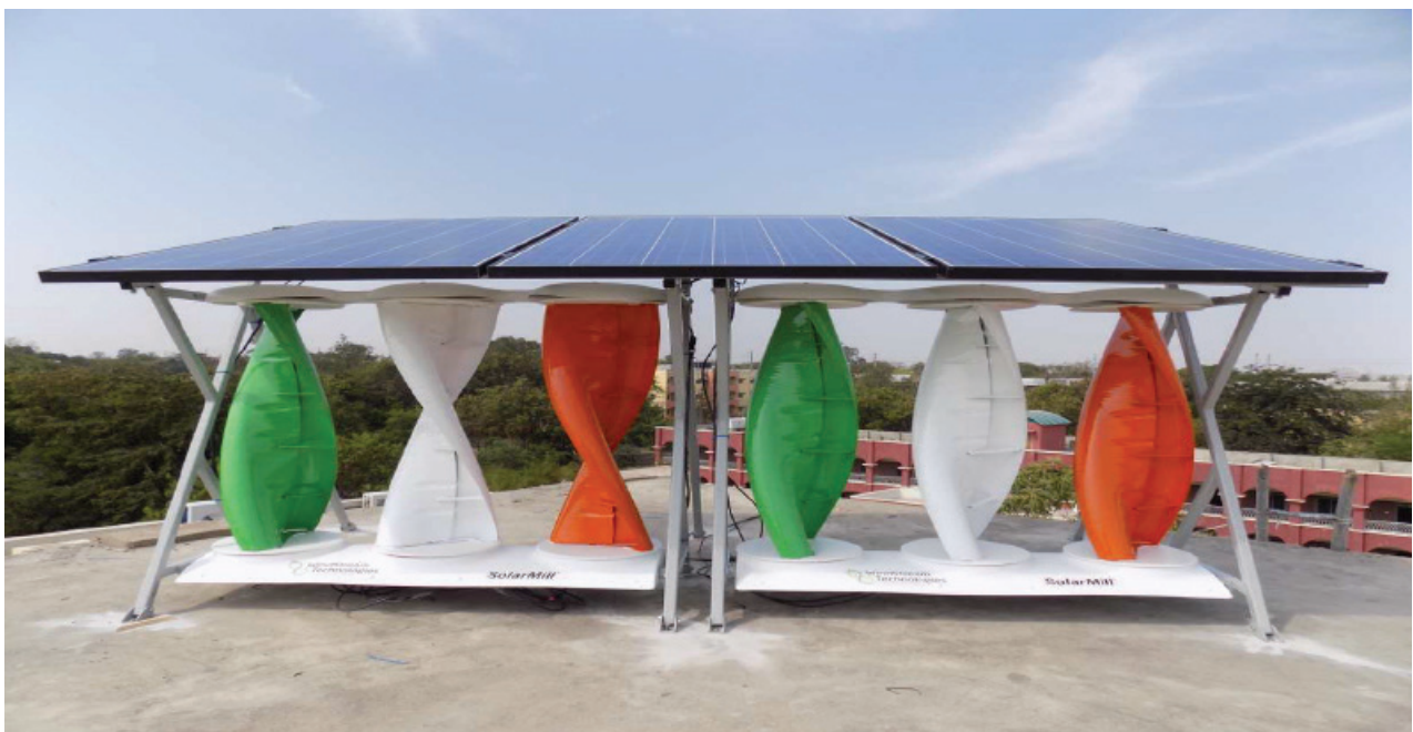
Figure 50: Solar wind hybrid system
