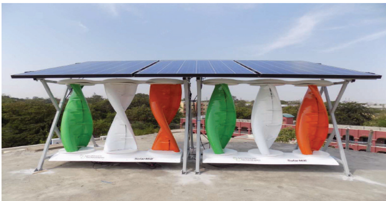
Figure 52: Solar wind hybrid system
