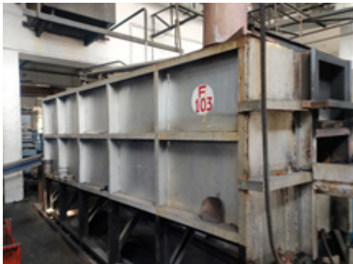
Figure 5: An oil fired reheating furnace
