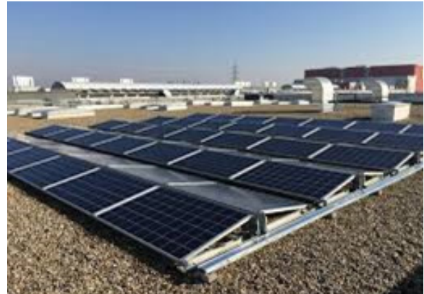
Figure 7: Solar PV installation
